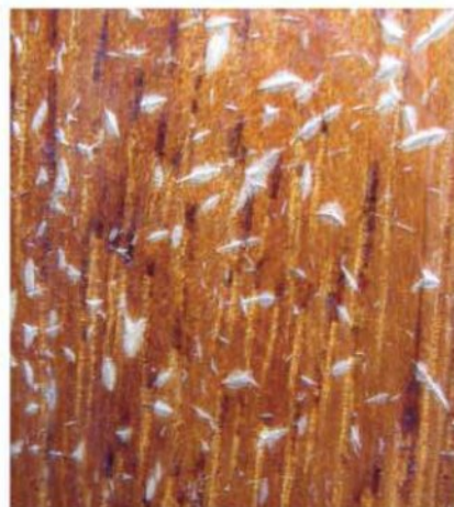
Looks can deceive - UV-Tech surface blistering, but it retains its integrity beneath.
